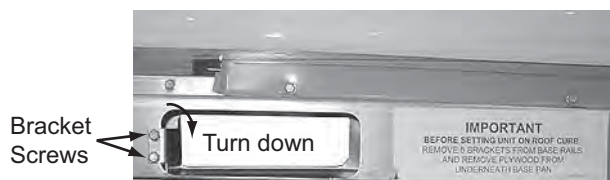
Figure 1: Unit Shipping Bracket
