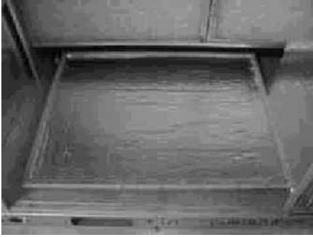
Figure 17: Return Panel In Place For Side Duct Conversion
